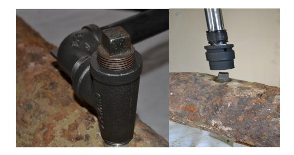
The process known to the gas distribution industry as "Service retirement" or "Service abandonment" for low- pressure (up to 10 PSIG systems) is a process that is performed on a cast iron gas distribution main. In these systems the service tees are threaded directly in the top or side of the main. Tellus has designed this procedure to be performed by two gas mechanics working in tandem to remove the service tee, plug the main and cap off the service line that remains in the ground.
