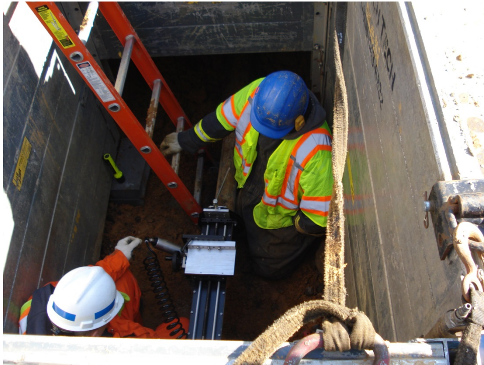
Window cutting machine: TAS-8034
