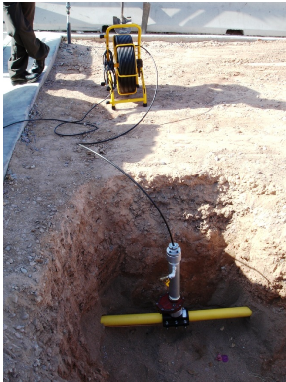
Stuffing box, Hathorn 1" camera: TCL-4201
