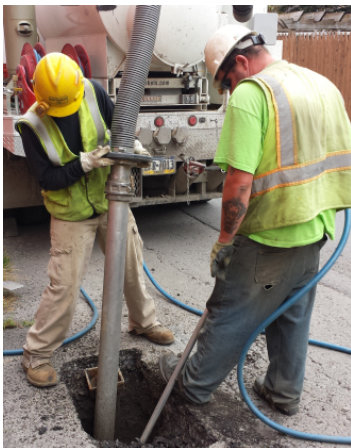
Digging tube head, 4" hose: TAS-8003
